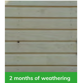
OFFICE SIDING, VROOMSHOOP, THE NETHERLANDS
