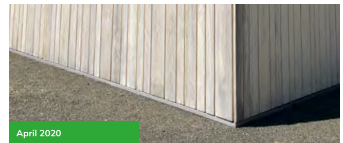
SIDING PROJECT, NORTH AMERICA
